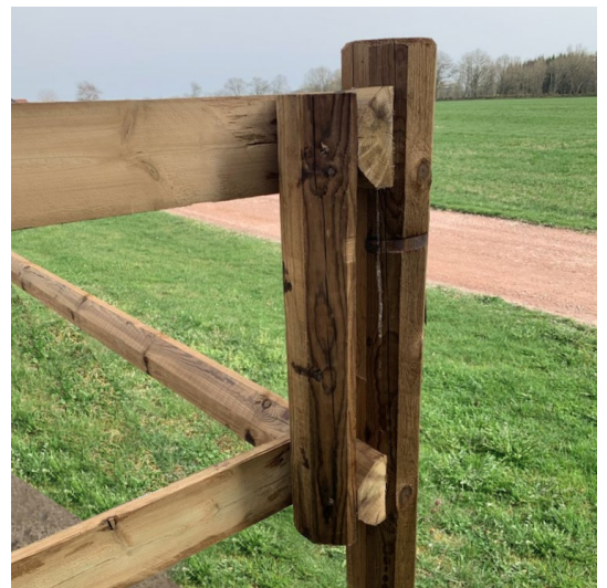
Picture 1: Corners for rails mounted on the inside of the paddock.
