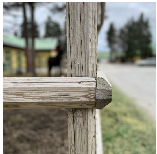
Picture 2: Corners for rails mounted on the outside of the paddock.
