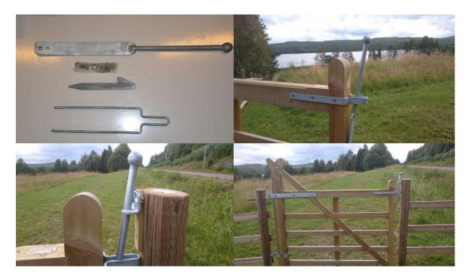
The cane bolt is mounted as shown on the picture. Remember that the higher the position of the gate above the ground, the lower the cane bolt needs to be mounted on the gate in order for the bolt to go far enough into the ground. Open the gate to the desired position and dig down the pipe so that it is positioned level with the ground directly beneath the bolt.
